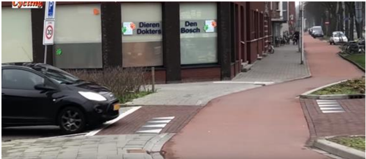
Figure 7: Raised Intersection between the bicycle lane and the road for motorized vehicles (Source: DutchCycling.nl)
