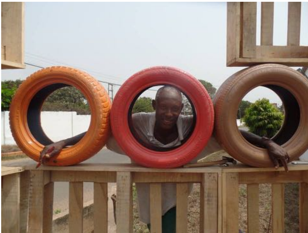
Image 11: Carpenter Mr Mensah during construction of the perimeter fence
