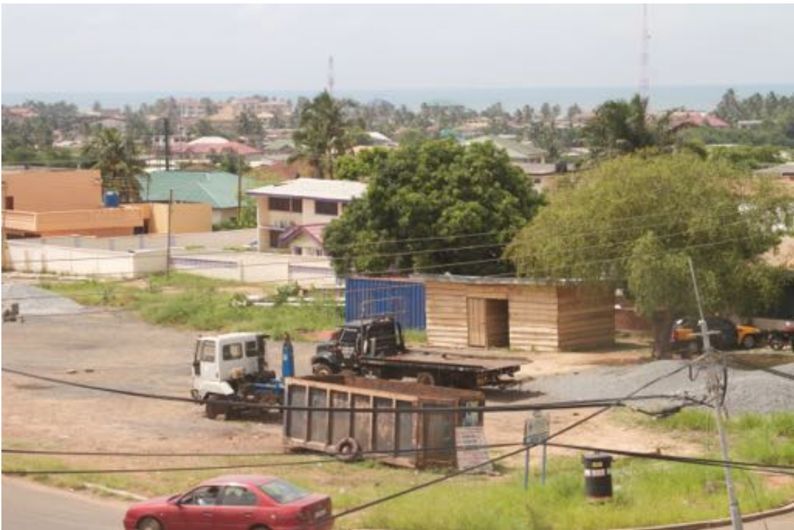
Image 17: Site before Intervention
