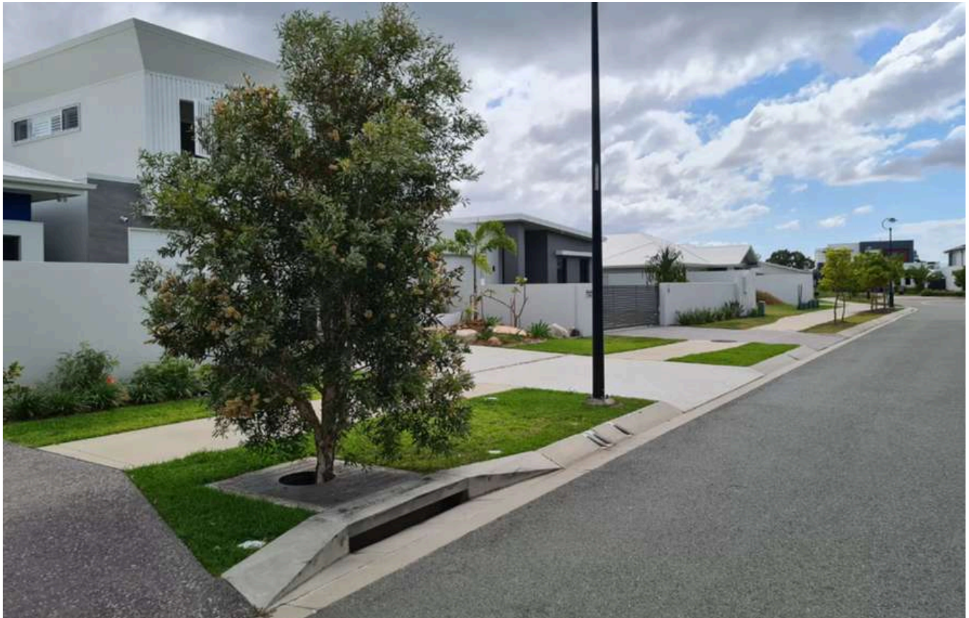
Integrated Design of Drainage and Street Tree Planting. Photo: Citygreen
