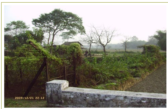
Figure 26: A gap in the fencing along the Indo-Bangladesh border
