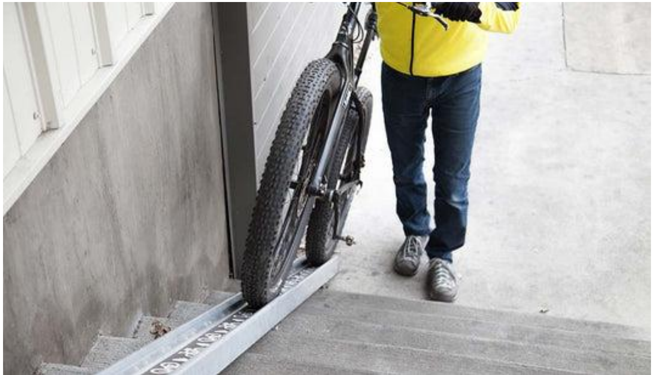
Figure 49. Bicycle access ramp installed on stairway
