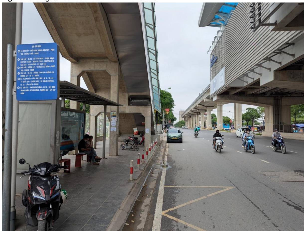
Figure 26. Singular transit shelter near Nhổn station
