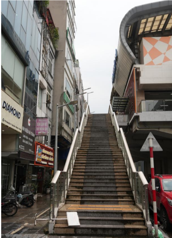
Figure 35. Exposed staircase at Thái Hà station
