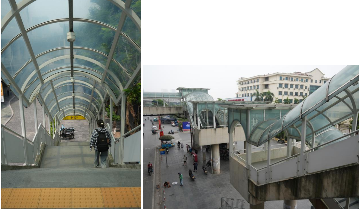
Figures 37 and 38. Glass canopies at National University station (left) and Nhổn station (right)
