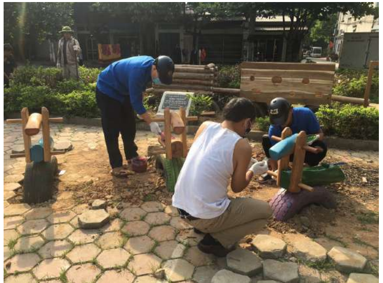
Construction of public spaces in Lao Cai
