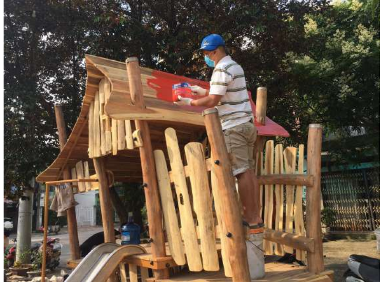
Construction of public spaces in Lao Cai
